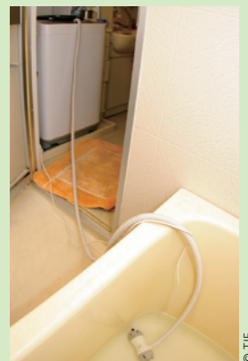
Hose and pump for recycling bath water for laundry.
